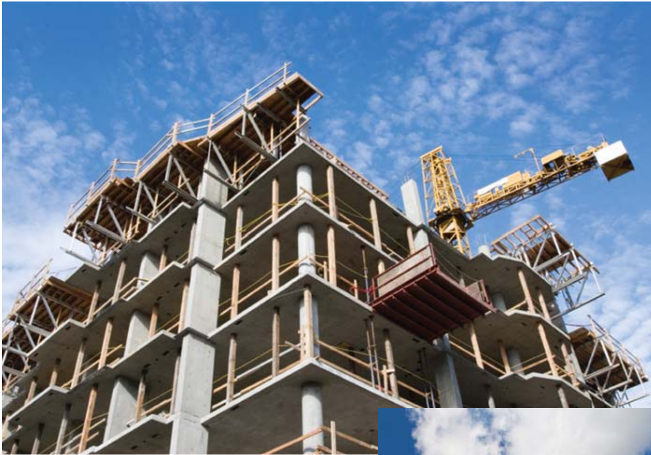
Construction Elevator Emergency Stops
